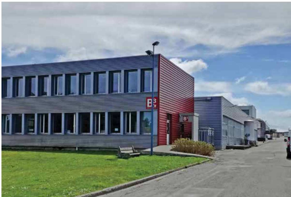
Our Plant in Lannion (FRANCE).
